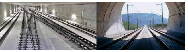
**The flexible way for all applications** The RHEDA 2000<sup>®</sup> ballastless track system is ideal for applications on embankments, on bridges, in tunnels, as well as for turnouts and with vibration-optimized mass-spring systems. Installation of noise absorbers attenuates noise from wheel-rail rolling and vehicle power-plant operation.
